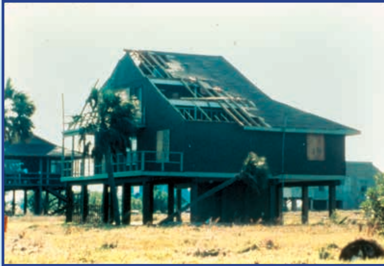
Above: Wind damage to home from Hurricane Alicia in August 1983.
