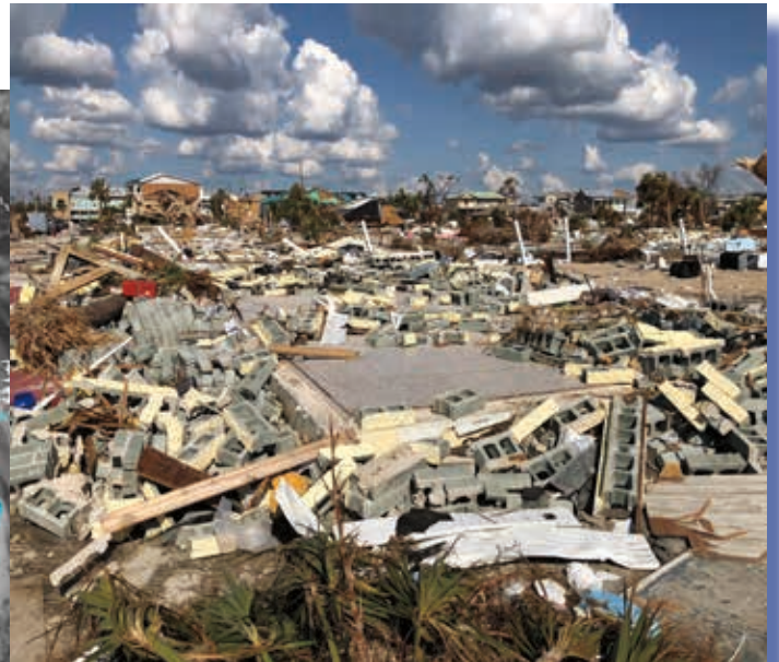
Damage from Hurricane Michael Photo Credit: Jeff Lindner
