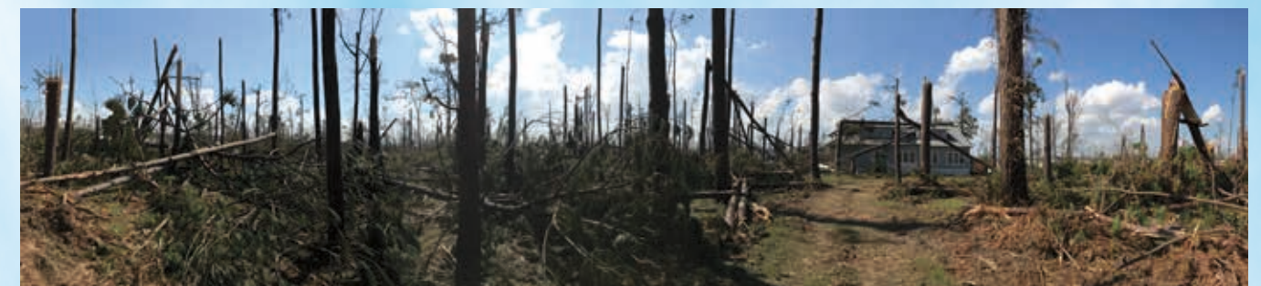
Figure 3. Photo showing tree damage near Lake Seminole, Decatur County, GA (well inland of landfall). Photo credit: Jeffrey Evans.
